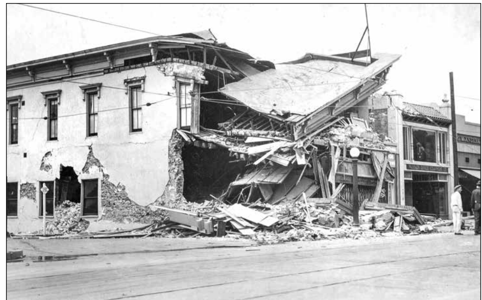
The 1925 Santa Barbara earthquake killed 13 people and caused millions in damages to downtown
